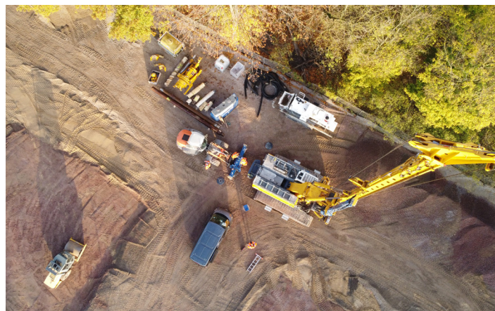
Havel Marina, Berlin - Installing the full displacement bored piles (STB Wöltjen GmbH)
