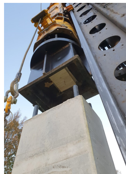
Handling pile into driving cap using special lifting device
