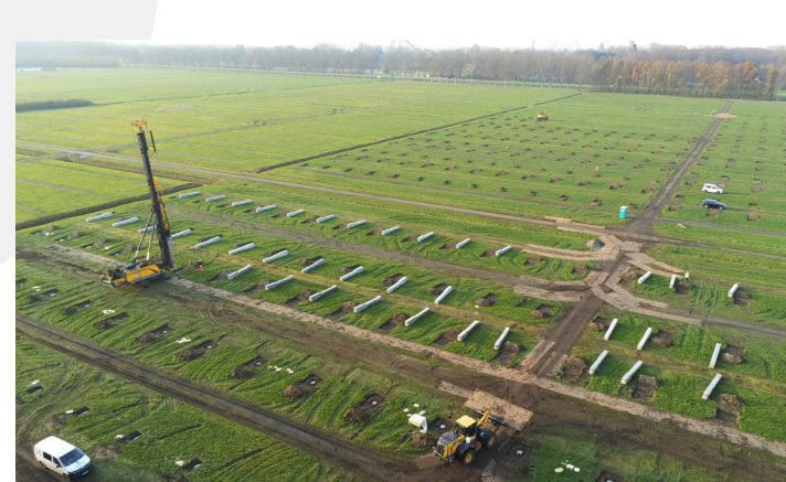
Centrum piles laid out to be installed at the MOJO site
