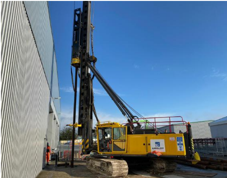
Driven Steel Tube, Gateshead - Piling Team
