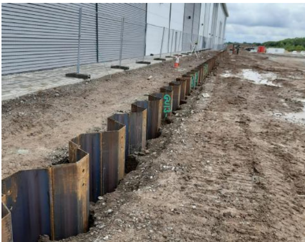
Sheet Piling, Manchester ICON - Jim Wilson
