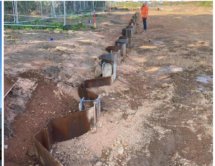
King Post Sheet Piling, Aberdeen - Jim Wilson
