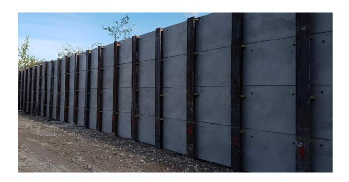
Aarsleff can design and construct King Post Walls for significant retained heights, very large dimensions and by different installation methods. They can be constructed as free standing cantilever walls, propped or as anchored structures offering numerous applications including basements, embankment and highway retention.
