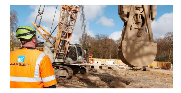
Diaphragm Walls are designed to reach great depth and provide the required structural capacity to facilitate certain construction activities such as retaining walls, underground structures, or as a form of foundation.
