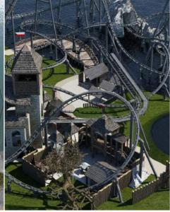
Chorzów Amusement Park, rebranded as "Legendia", boasts the largest rollercoaster in Central Eastern Europe. The ride reaches a height of 40m, has a maximum speed of 95kph, and has a track length of 908m. The ride also features three inversions. The structure was designed to have 187 foundations, with 12 types of foundation solutions.
