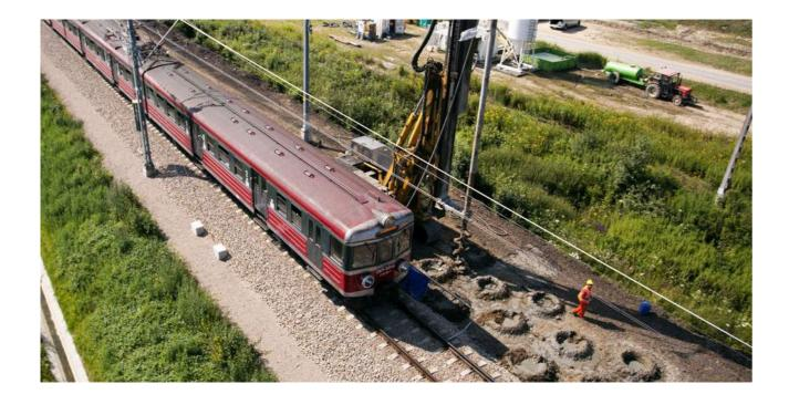
Ground Improvement methods are used to improve the existing soil formation by changing the soil properties. They can increase the bearing capacity, provide settlement control for new construction, or remedy an existing issue.
