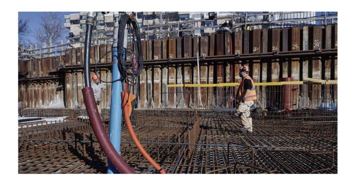
When a client is to build in an area with a high water table, it might be necessary to carry out Groundwater Lowering in order to prevent significant groundwater seepage into the excavation and to ensure stability of excavation side slopes and base.
