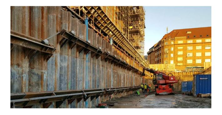
Aarsleff's in-house capabilities enable it to design, supply, install & extract Sheet Piles whether for temporary or permanent works. Sheet piles can be used for a variety of applications including cofferdams, retaining walls, seawalls, bulkheads, access jetties or other applications where earthworks support is required. Additional support can be provided via hydraulic or in-situ frames, tie-rods or anchors.
