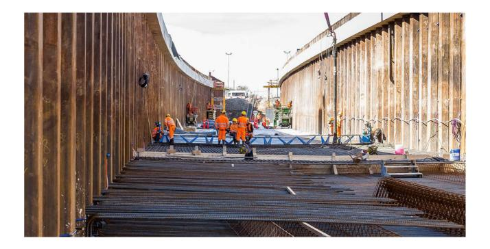
Construction Pits/Cofferdams will most often consist of a relatively impermeable wall built around the periphery of the proposed excavation. Sheet pile walls are widely used in construction pits, but secant piles, diaphragm walls and other structures can also be used.
