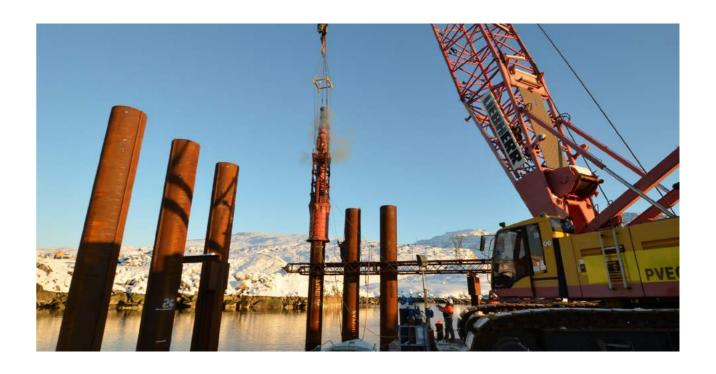
Steel Piles, such as tubes and H-Sections, are usually installed for marine structures or as foundations for temporary structures, permanent bridges, acoustic screens and buildings with underground floors. Depending on soil conditions, Aarsleff can install steel piles using two technologies - or a combination of both:
