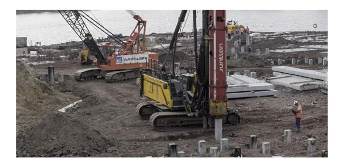
Along with the installation of 39No. precast piles with various cross-sections, lengths and reinforcement, Aarsleff both constructed and disassembled access roads and a temporary working platform on land and in water, using 17,800 t of red-burnt shale. They also constructed monolith pile caps for 12 foundation types as well as performed 22No. dynamic load tests.
