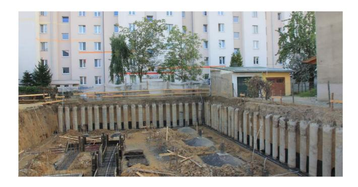
Aarsleff Ground Engineering has the specialist plant and team to install Contiguous Pile Retaining Walls. The walls are constructed with nominal gaps between adjacent piles, depending on retained heights, installation tolerances and allowable deflections.
