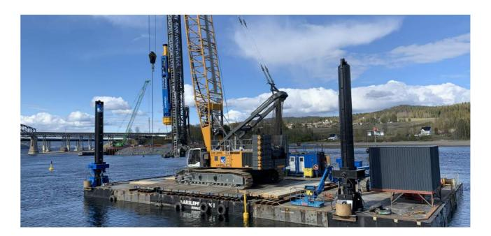
The foundation of the Minnevika bridge consisted of 268No. driven piles in total, all with a diameter of 1016mm and installation lengths of up to 58m. All piles were set out in a tight scheme, thus arranged with an inclination of 1:10 - 1:5 in order to resist ice loads, brake forces etc. In addition to the piling works, Aarsleff also installed 17 cofferdams (up to 20x24m²) using sheet piles with a length of 19m allowing for excavation to a depth of approx. 10m.
