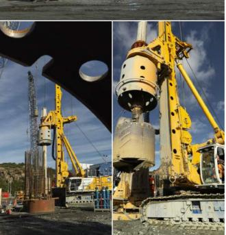
tool was replaced, and drilled up to seven metres into the rock, depending on the location and function of the pile. The casing pipe was constantly filled with water to protect against heave in the pile during production. After completion of the drilling work, the hole was cleaned by means of airlifting, and the reinforcement was lowered down into the casing pipe. To optimise the installation, the reinforcement was mounted in advance in three installation pipes driven 30m into the around.
