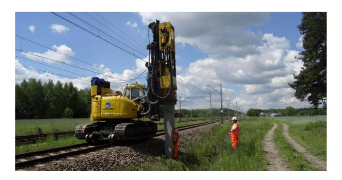
Mast Foundation Piles are precast piles specifically designed for the masts of the railway electrification system, as well as special anchor piles. They are driven with a special rig, able to move on railway tracks and equipped with a hydraulic hammer; the frequency and height of which are electronically controlled. The machine can also safely work under the existing electrification system.
