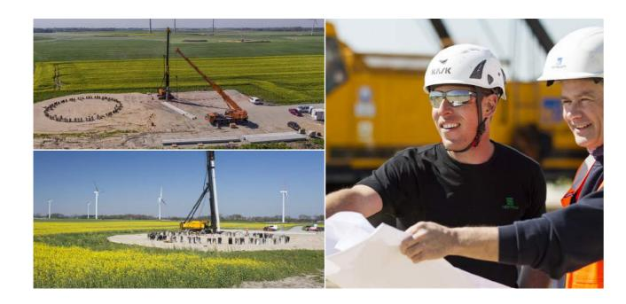
Aarsleff was appointed to install the pile foundations for wind turbines including foundations for the assembling crane at the Wetterdeich wind farm in Lower Saxony. 7 WEA of the type ENERCON E-115 were built for Bürgerwindpark Oederquart GmbH and Denker & Wulf AG.
