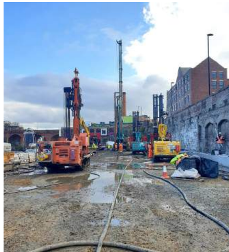
Drilling & Grouting, Ouseburn - Phillip Wright
