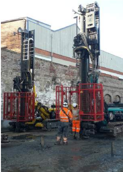
Drilling & Grouting, Ouseburn - John Waugh
