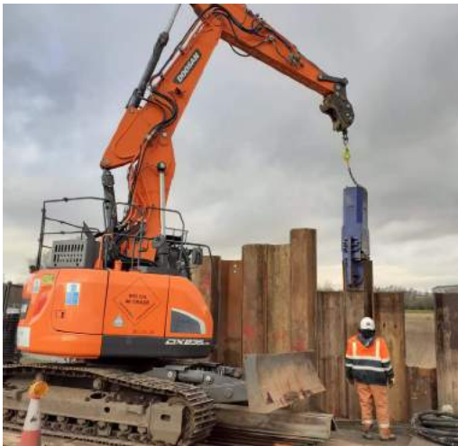
Sheet Piling, River Doe Lea - Jim Wilson
