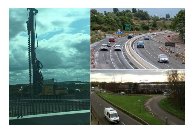
Scope of Works 223 lin/m steel pile retaining wall 372No. steel sheet piles Pre-auger at 600mm
