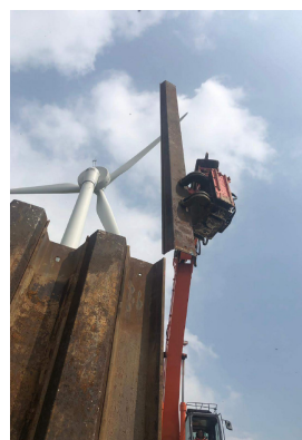
Sheet Piling, Kings Lynn - Vasil Dilov
