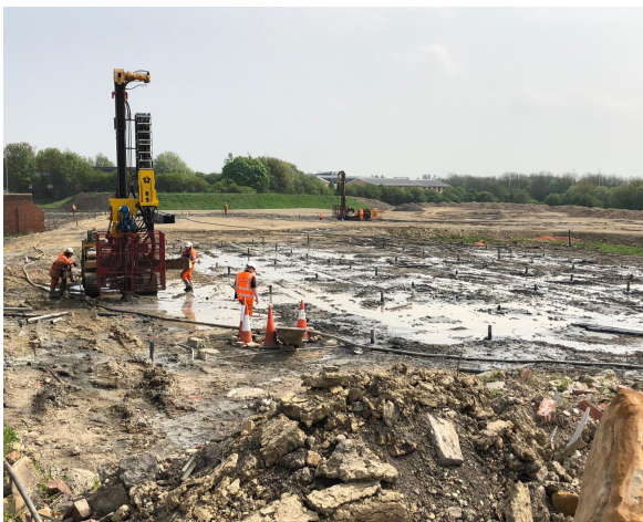
Drilling & Grouting, Gildersome - Chris Purvis
