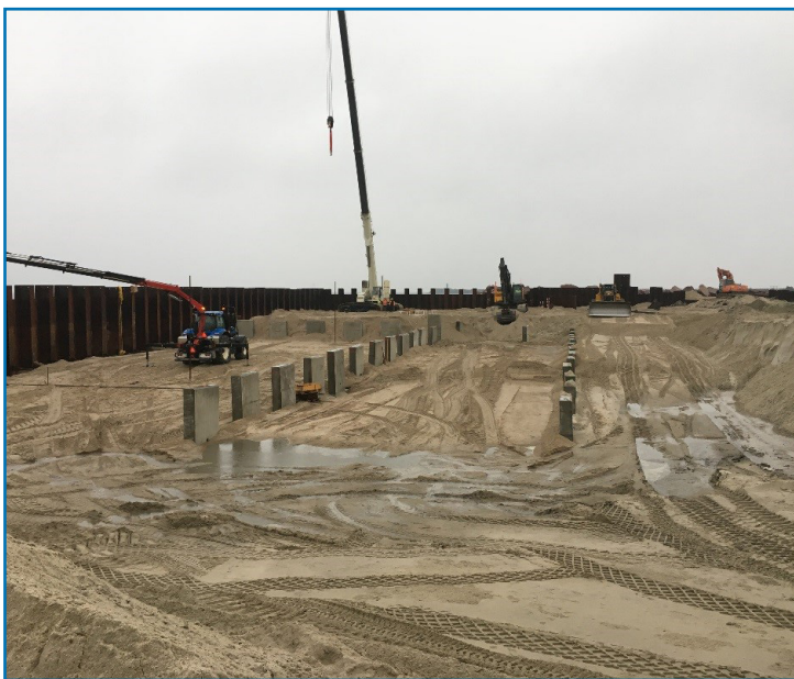
Figure 6: Anchor plates placed 23m or 35m in land.
