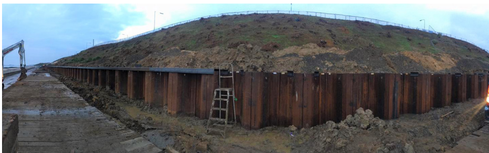
Sheet pile wall with capping beam, Clacton on Sea - Joseph Mills
