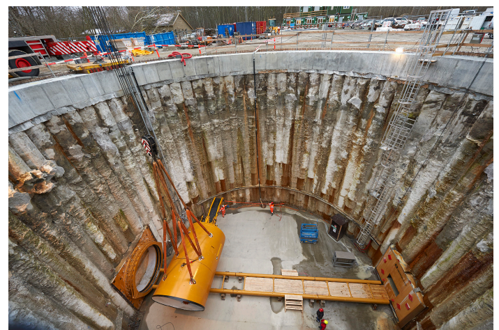
Secant Pile Wall - Per Aarsleff A/S
