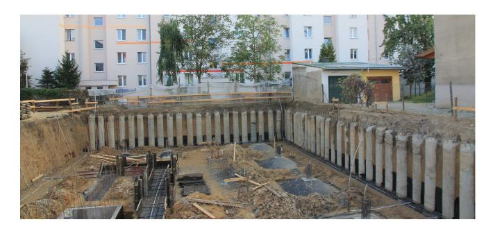
Aarsleff Ground Engineering has the specialist plant and expertise to install contiguous pile retaining walls. Contiguous pile walls are constructed with nominal gaps between adjacent piles, depending on retained heights, installation tolerances and allowable deflections. The gap between each pile is typically 150mm. These can be constructed to provide load bearing capacity as well as a retaining
