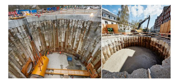
Secant bored pile walls are formed using interlocking primary and secondary piles. The secondary piles are first installed with the primary pile cut in to the secondary pile. The secondary pile can be described as soft, firm or hard depending on the design requirements. A soft and firm pile resists the loss of ground between the structural piles along
