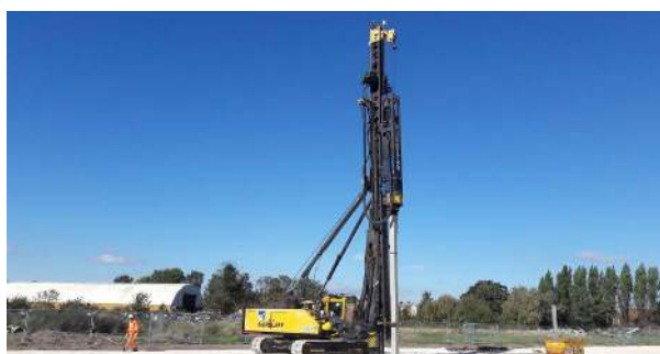
Precast Piling, Port of Boston - Sam Riley
