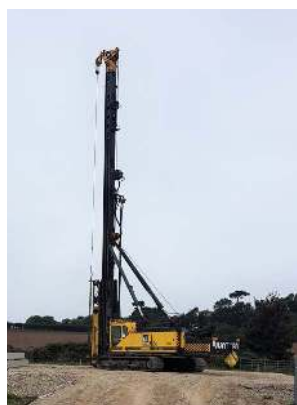
Precast Piling, Richborough - Stuart Hancock
