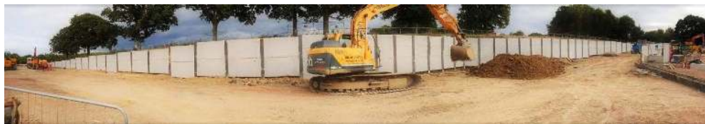
King Post Wall, Goddards Green - Jim Wilson
