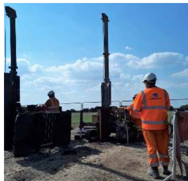
Bottom Driven Piles, Richborough NG Connection - Richard Judd
