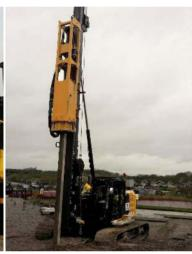
Aarsleff commenced on site in early September 2018, installing 303No. precast concrete piles with its Banut 300 rig, ideally suited for restricted access sites. The piles were 250mm square section and between 5-13m in length, designed to cater for up to 455kN compressive working loads. All piles were manufactured in Aarsleff's sister manufacturing facility Centrum Pile and were therefore tested and confirmed as structurally competent before delivery to site.
