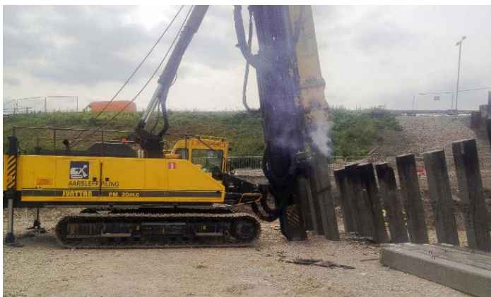
Figure 3. Raking precast concrete piles being installed with a hydraulic impact hammer
