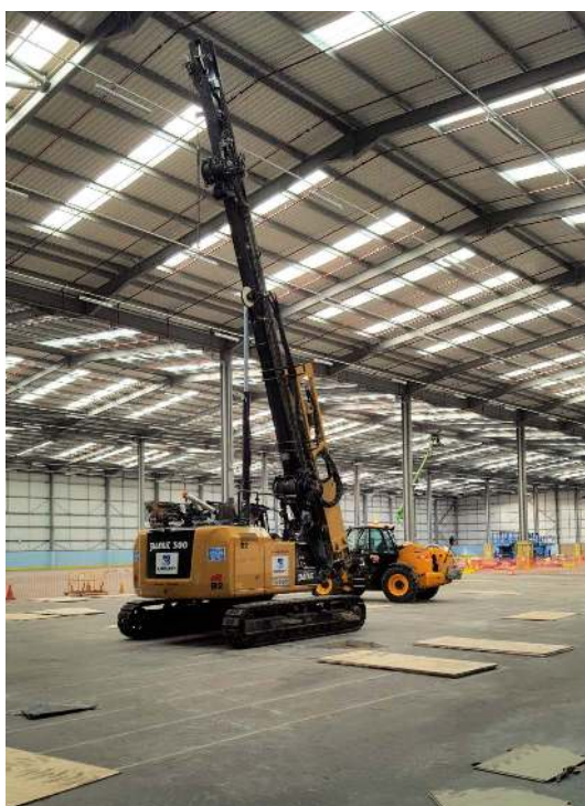
Precast Piling, Hatfield - Simon Cottington
