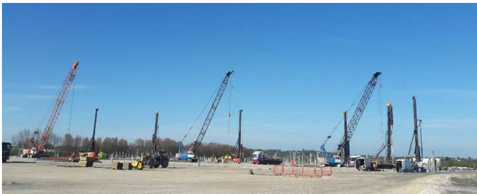
Driven Precast Piling, Eastwood - Parth Patel
