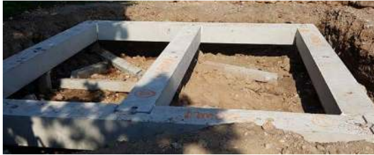
Ground Beams, Stoke on Trent - Phillip Hall
