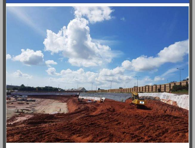
Aarsleff Ground Engineering were awarded the contract to supply and install the soilnailed wall required to support excavations to allow the construction of a new IKEA in Exeter, just off Newcourt Way near Sandy Park.
