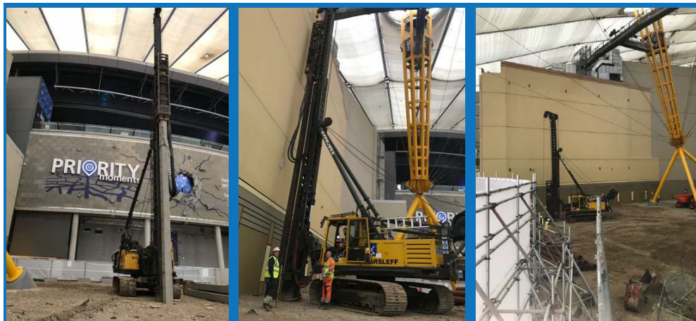
Piling inside the O2 Dome, London - Lee Severn
