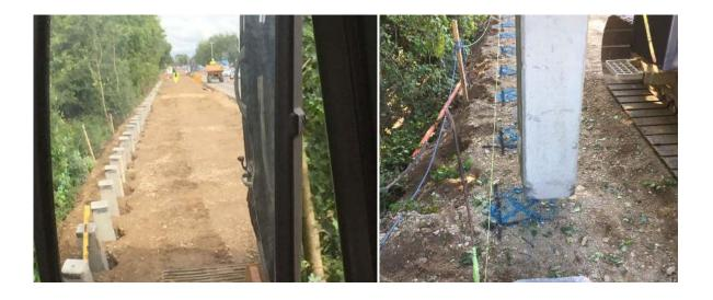
Scope of Works 300 No. 300mm Driven Precast Concrete Piles
